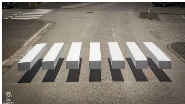
Figure 10: Experimental 3D Crosswalk Marking Pattern (Iceland)
