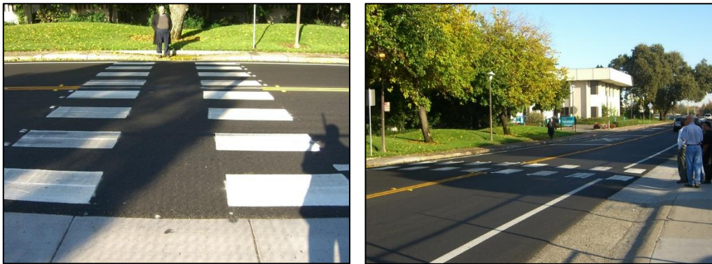
Figure 7: Example of "Triple Four" Crosswalk Pattern
