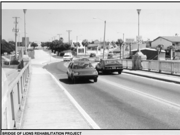
BRIDGE OF LIONS REHABILITATION PROJECT
