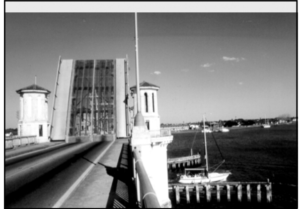
BRIDGE OF LIONS REHABILITATION PROJECT
